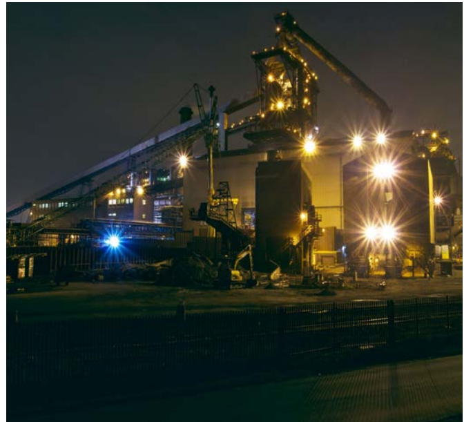
Impianti Industriali / Industrial Equipment / Industrieanlagen
