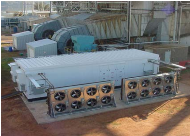
Example of installation with W32 option (advanced cooling cabinet): There are two water-cooled drives in the building
